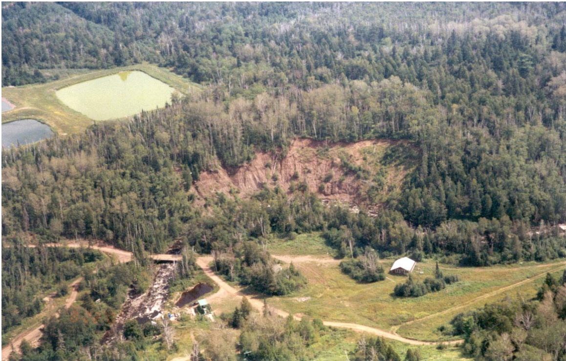
Figure 26. Eroding stream bank in the Poplar River Valley (note wastewater ponds in background)
