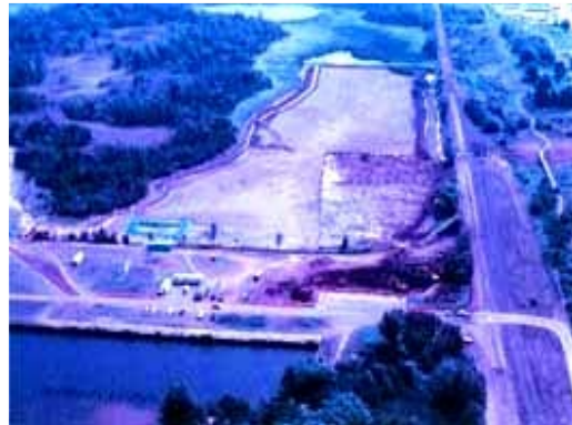
The Inlet was drained to be able to remove petroleum-contaminated sediment. (photo: USEPA Great Lakes)
