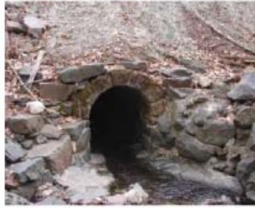
Entrance to the 4' x 5' Brick Arch Tunnel under 4 th St at 22 Ave E
