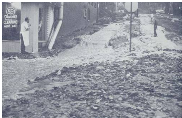
Clarkhouse Cr. below Cascade Park along First Ave. West
