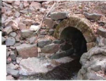
Entrance to the 4' x 5' Brick Arch Tunnel under 4 th St at 22 Ave E
