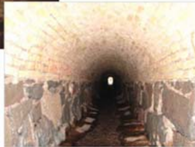
Oregon Creek 4' x 5' Brick Arch Tunnel at 4 th Street
