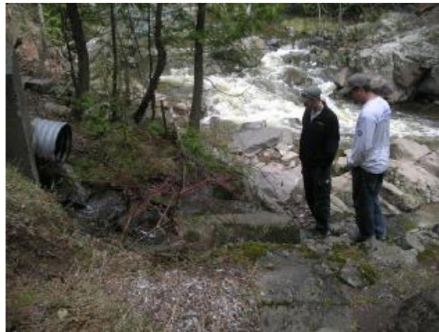
Figure 5: Storm drain entering Amity Creek.
